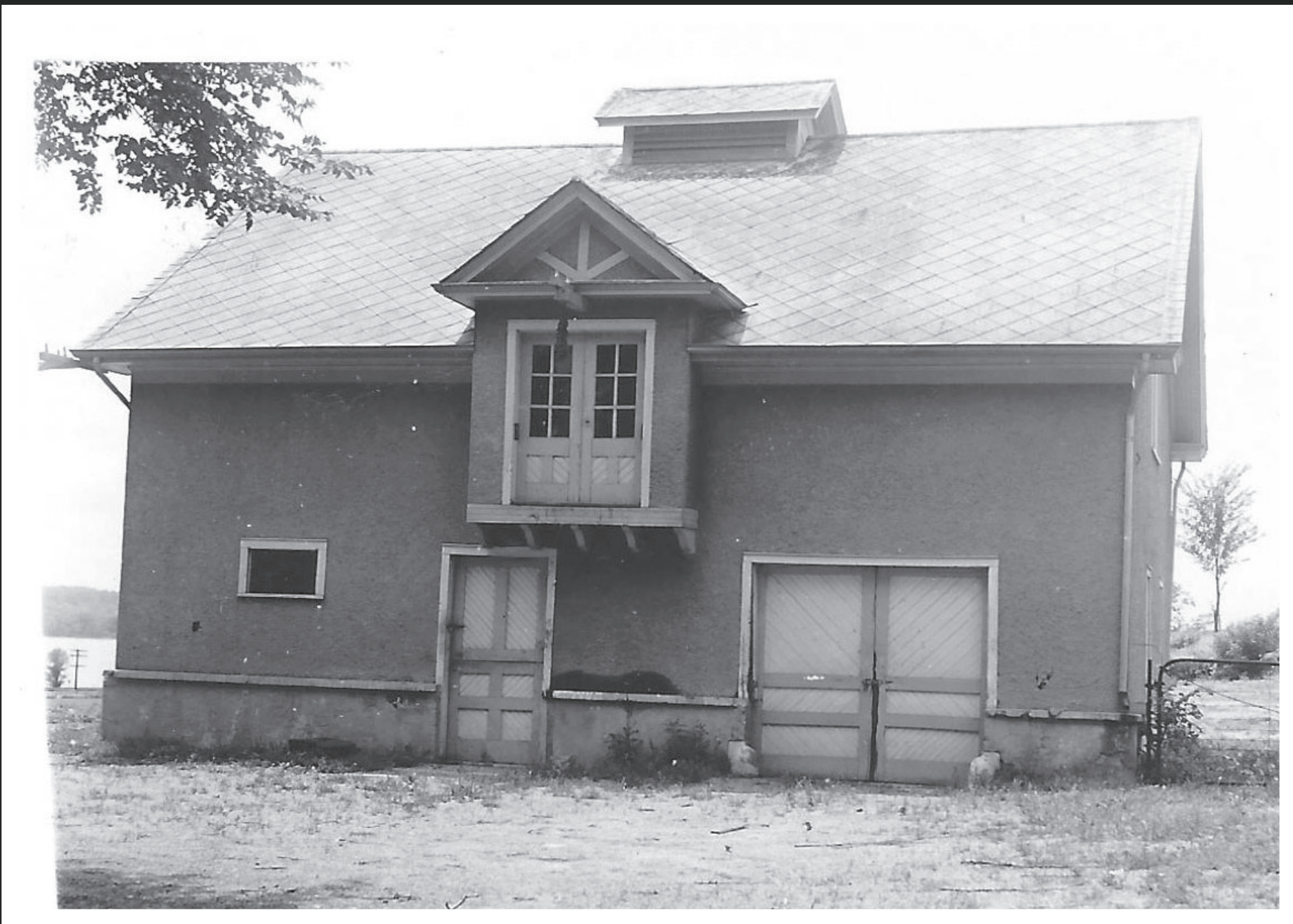
Overview of Barn in 1941 (note the stucco exterior), facing west.
