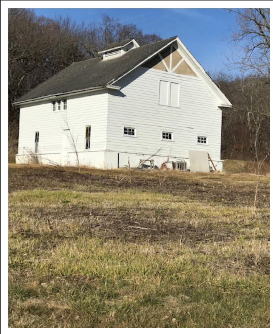
Overview of Barn in 2020, wood siding has replaced stucco, facing north. Note: Original pebble-dash stucco can be seen in the gable between the decorative stickwork.
