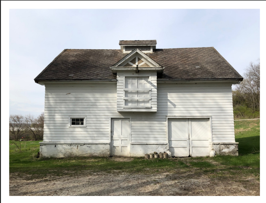
Overview of Barn in 2021, note wood siding has replaced stucco, facing west. Note: Original pebble-dash stucco can be seen in the gable between the decorative stickwork.
